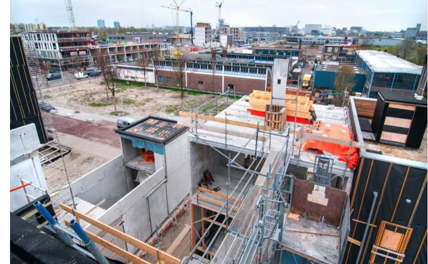
Circular construction - Amsterdam
