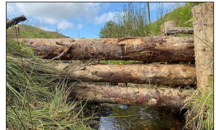
Log leaky dam
